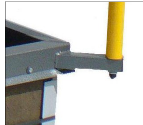
Rail Supports are Welded to Curb
